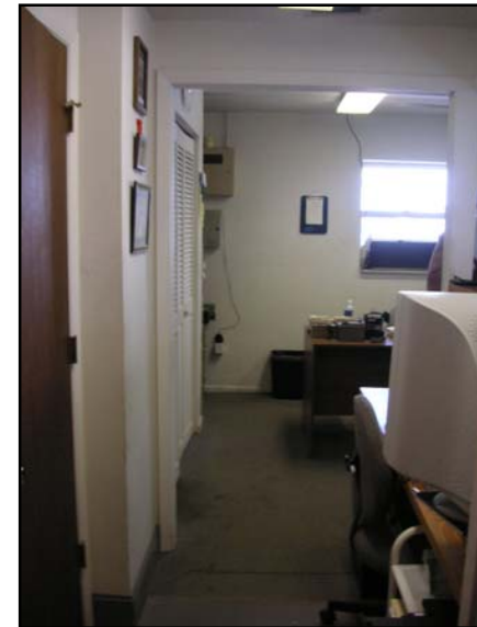
Office: Prior to Renovations
